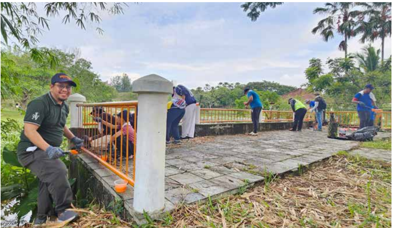
Beautification of Public Spaces: We undertook the revitalization of lakeside gazebos, restoring these shared structures to enhance the quality of life for the community.
